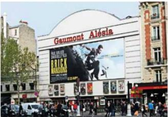
centre of the screen, the panels are glazed and covered with bars of LEDs while on the edges of the facade, the panels are built of metal cladding to make them opaque. Then they're either covered with the same LED-coated bars as the middle of the panel, or just pleated to "reproduce the rhythm of the LEDs."
