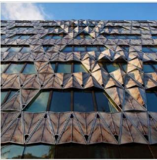
A variety of effects are created through the "folded" panes with stone-like film application: depending on the angle of the sun's rays, the color of the material as well as the play of light and shade vary.
