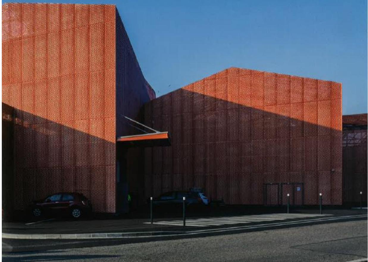
The roof of each volume is then systematically made of two slopes, inspired by the design of the roofs you can observe in the surroundings, alternating the orientation of the folded faces sometimes north-south, sometimes south-west, in order to capture a light each time different. The expanded metal, used as a cladding on all the facades, also contributes to this unity, and gives the project its originality.
