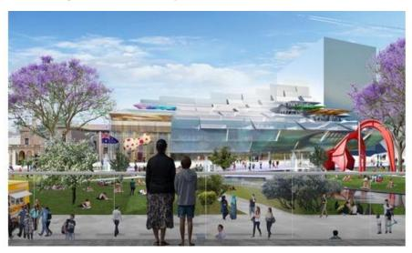
According to the development application, the building will form part of the greater Parramatta Square redevelopment and comprise six levels above ground with a sloping glass façade on the southern side, and a basement level with a partial mezzanine.
