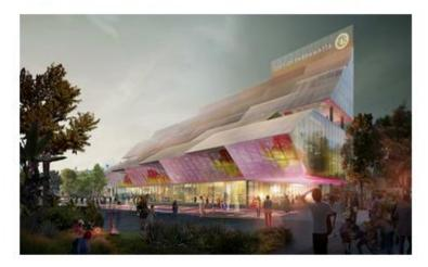
The façade to level one will be glazed with an integrated LED screen with lines of LEDs which will be stretched along the whole south façade, from the existing town hall to the south eastern corner.
